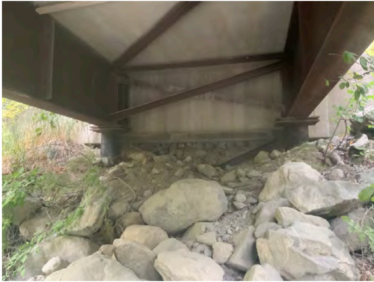
Right Bank Abutment when facing downstream
