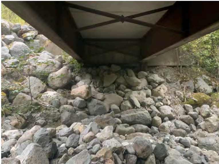
Left Bank Abutment when facing downstream
