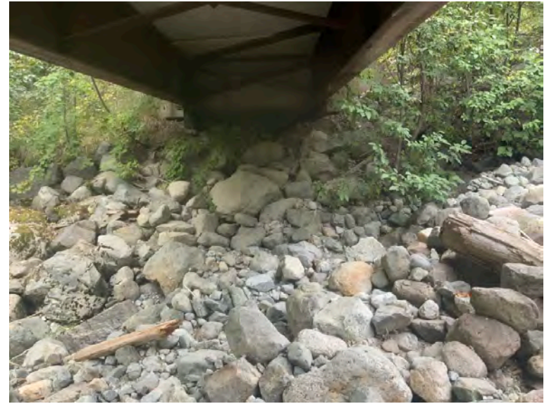
Right Bank Abutment when facing downstream
