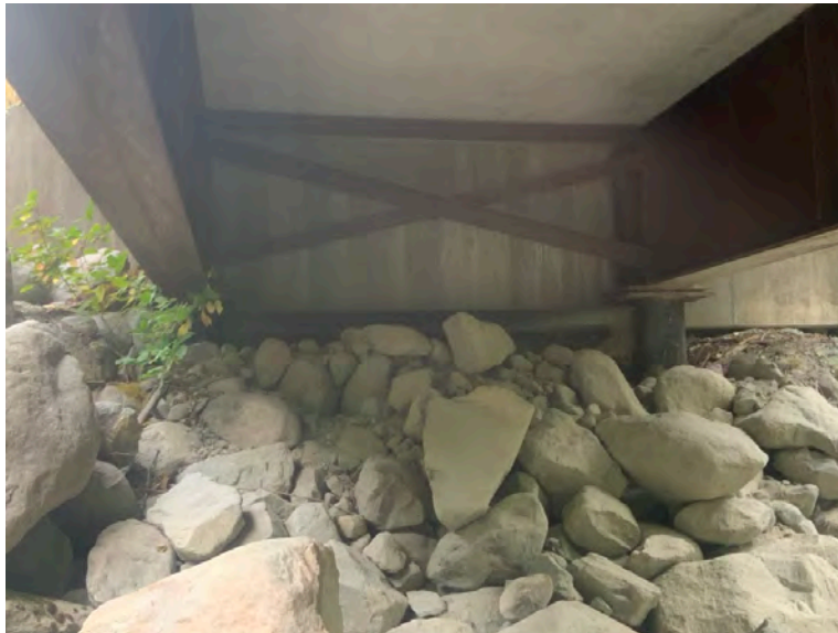
Left Bank Abutment when facing downstream
