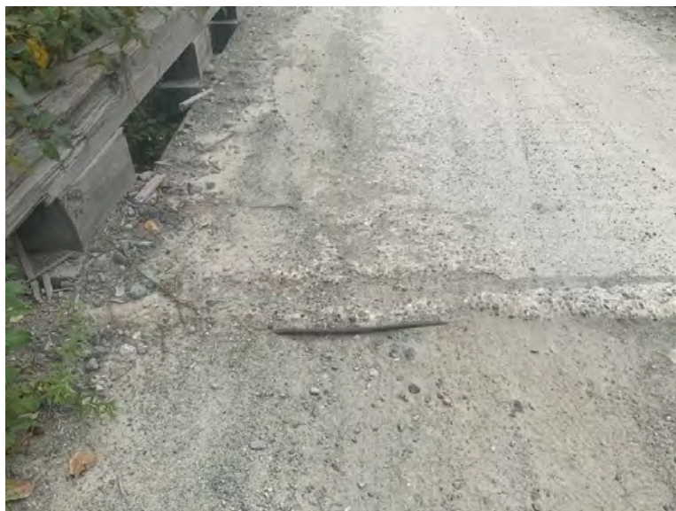
Deck, ballast wall. Town approach
